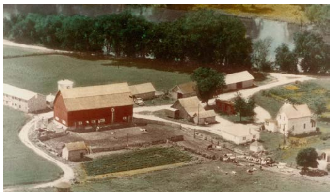
IMAGE 15 | Becker farmstead site adjacent to the Crow River circa 1953
